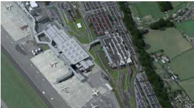
Computer generated image of the completed MSCP2/PTI with bridge link allowing direct access to the Terminal
