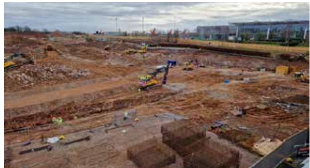
MSCP2/PTI under construction on the site of the former Long-Stay carpark
